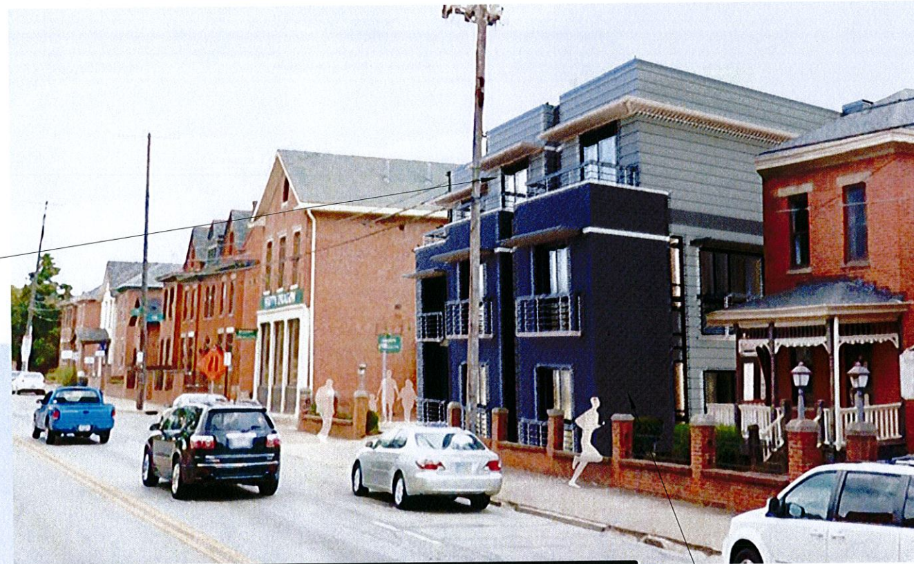
VIEW EAST @ E. LIVINGSTON AVE.
