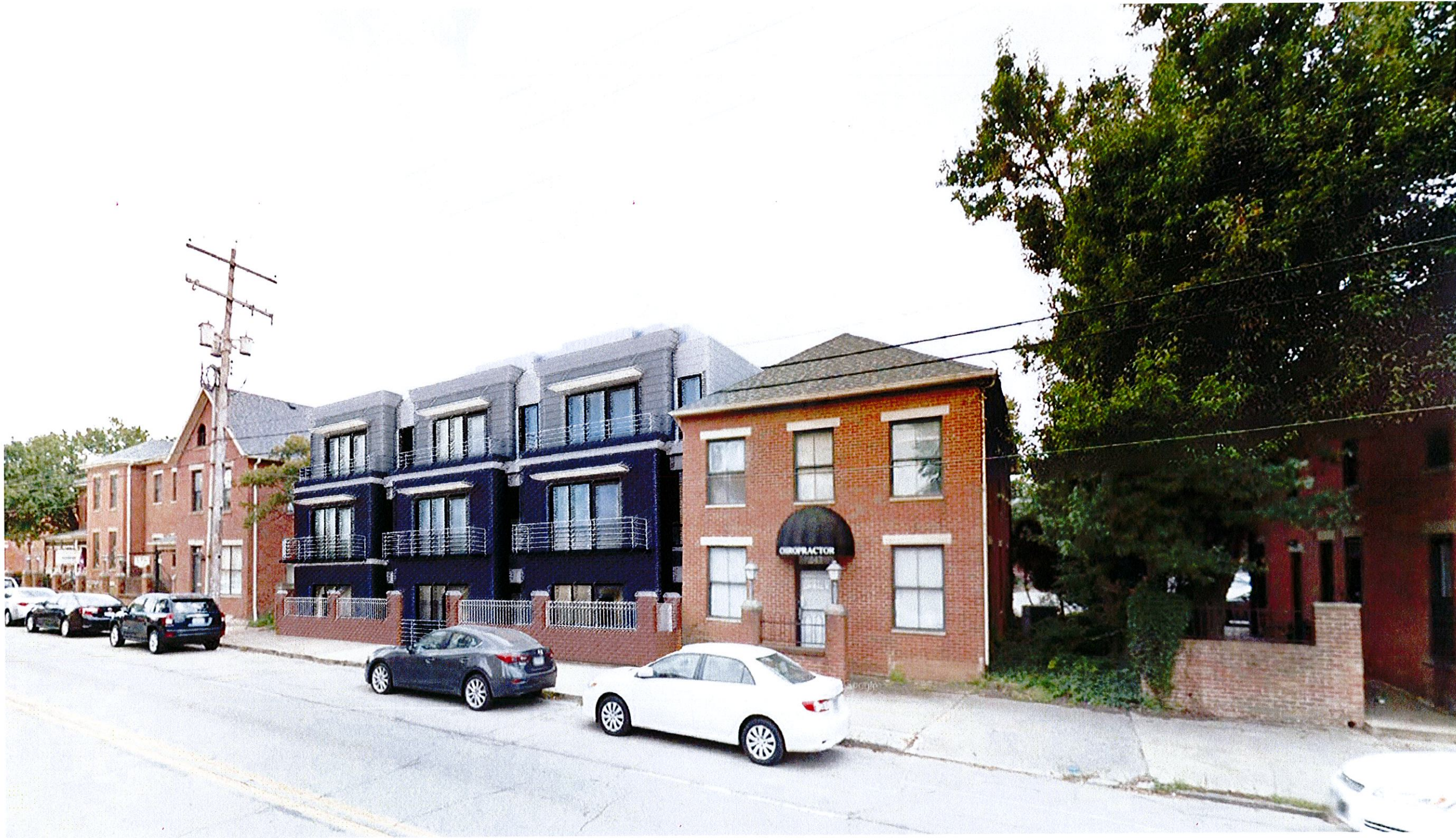
VIEW EAST @ E. LIVINGSTON AVE.
