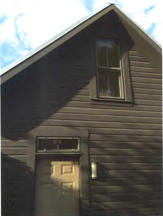
SOUTH FACING WINDOW-BACK YARD
